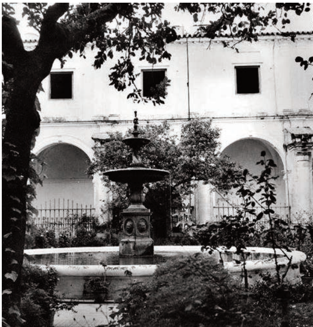
Patio Hospital Santa Isabel
